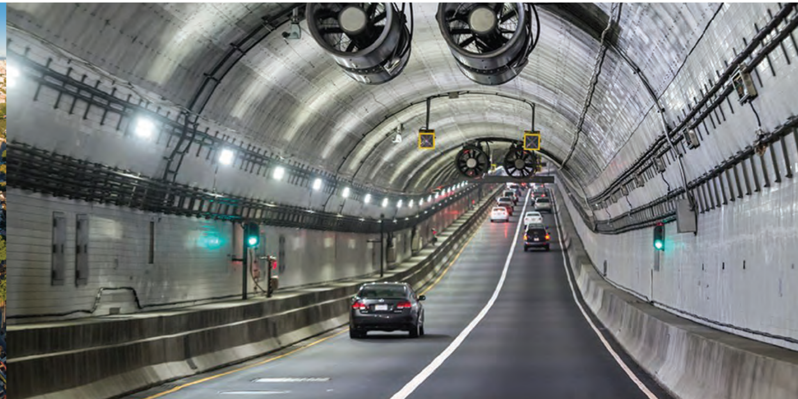
Abertis EEUU Elizabeth River Crossings
