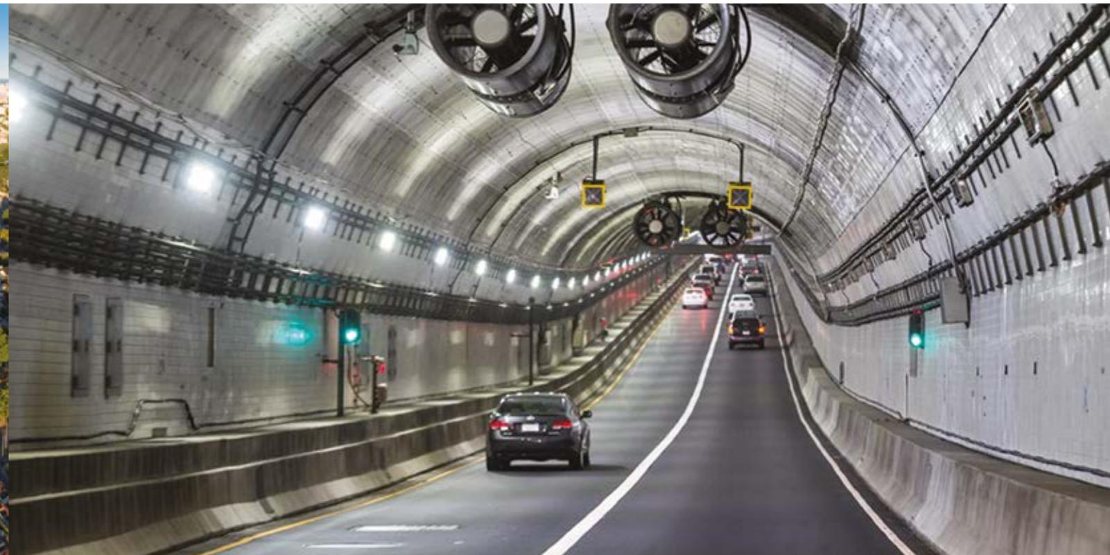
Abertis EEUU Elizabeth River Crossings
