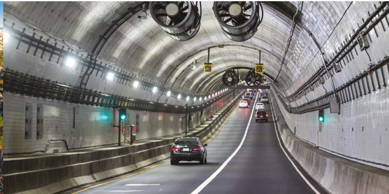
Abertis EEUU Elizabeth River Crossings
